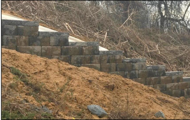
The new retaining wall near 3116 Lawrin Court will help stop erosion.
