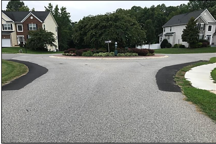
Traffic circle gets asphalt repairs.
