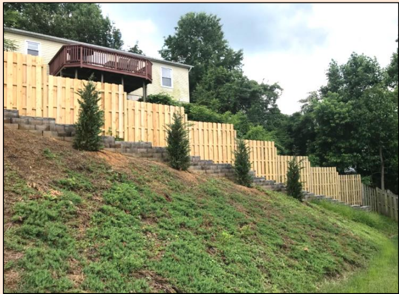
The new fence near 3116 Lawrin Court.
