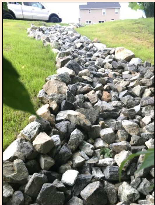
The rip rap near 3122 Lawrin Court.
